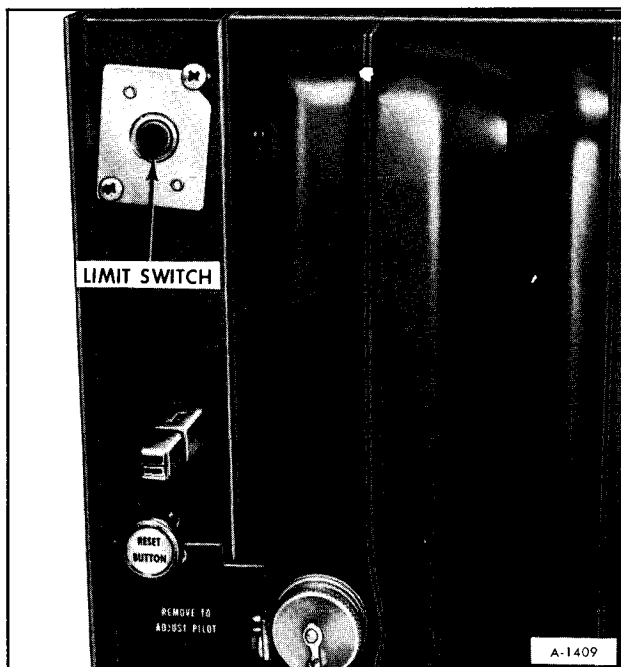
Figure 43—Type II Furnace Limit Switch
