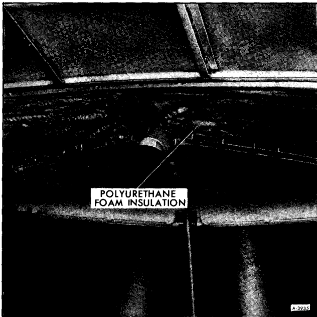
Figure 37—Cab Roof Insulation
