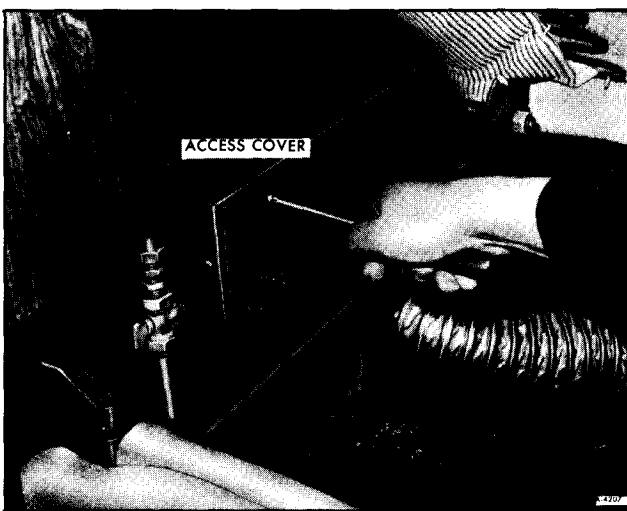
Figure 11—Removing Furnace Access Cover
