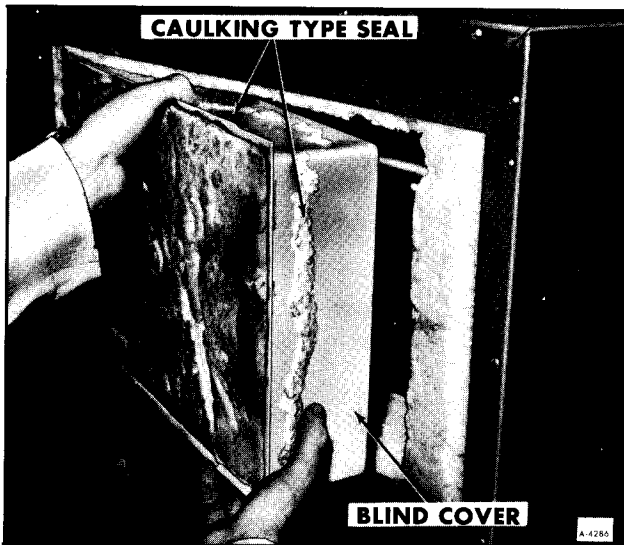
Figure 15—Removing Blind Cover
