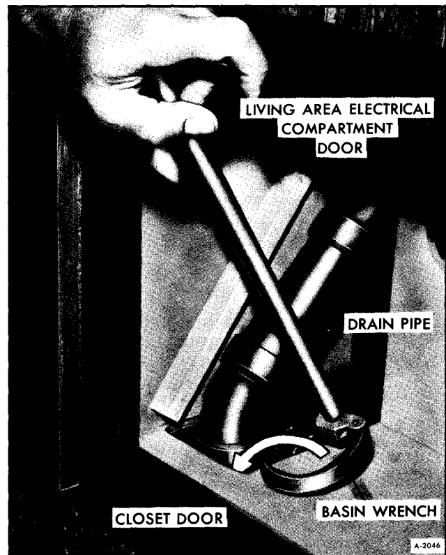
Figure 3—Loosening Pipe Fitting
