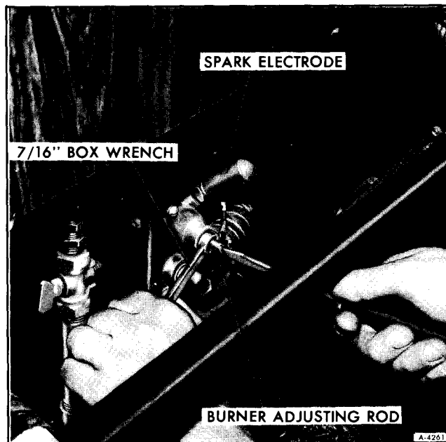
Figure 31—Furnace Primary Air Adjustment
