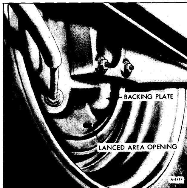
Figure 6—Lanced Area in Backing Plate
