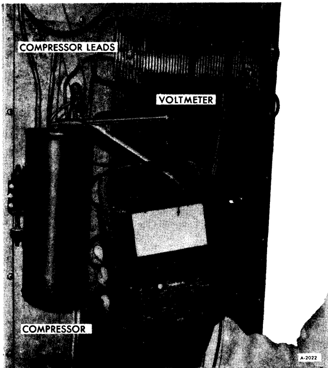
Figure 1—Checking Compressor Voltage
