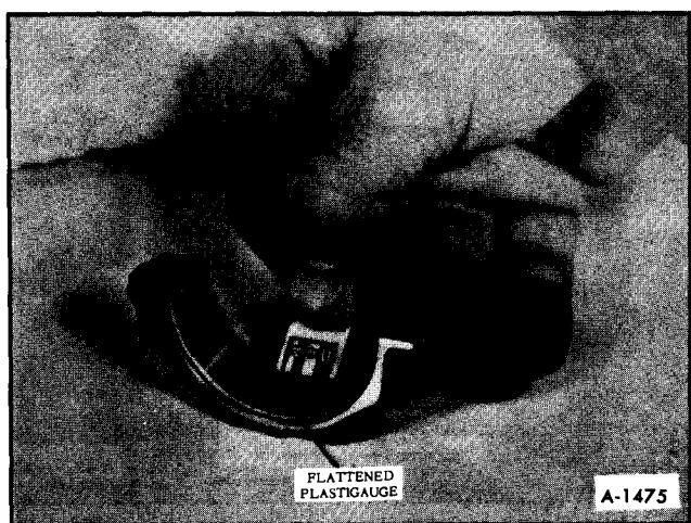
Figure 69—Checking Bearing Clearance
