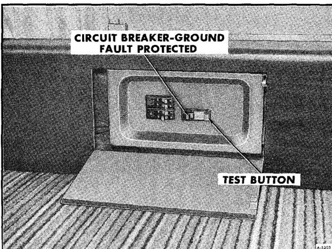
Figure 2—Circuit Breaker Panel (Model ZEO6582)
