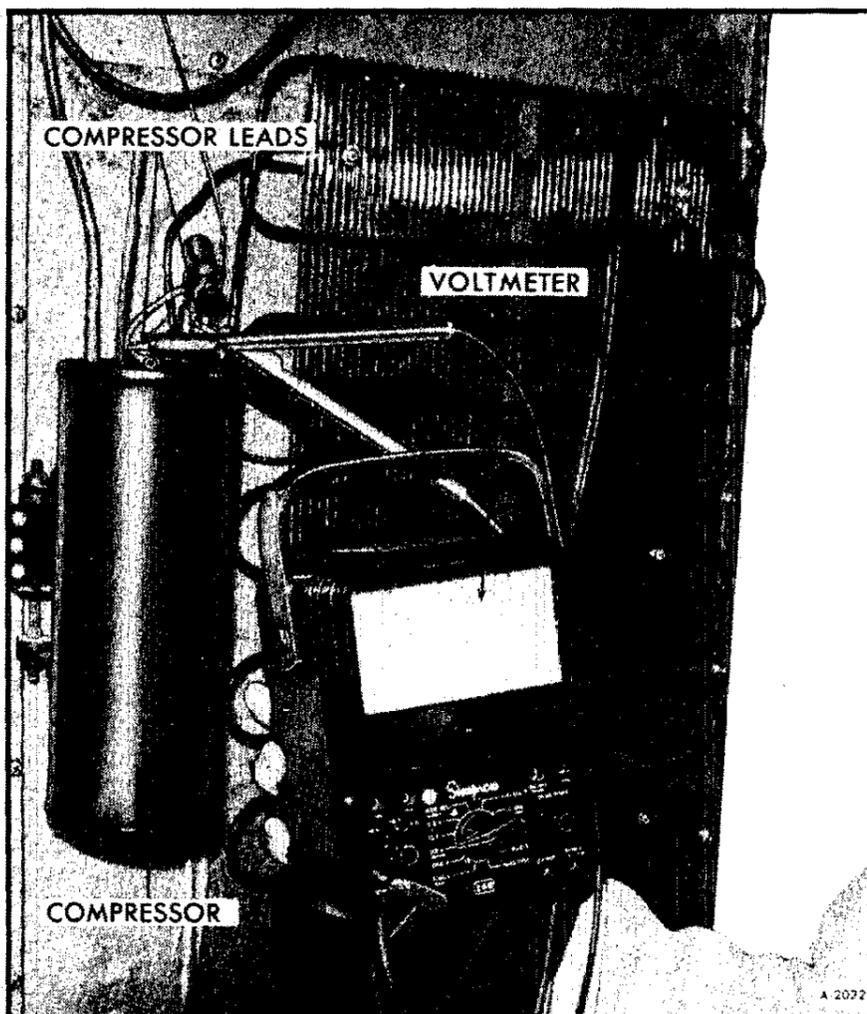
Figure 1—Checking Compressor Voltage
