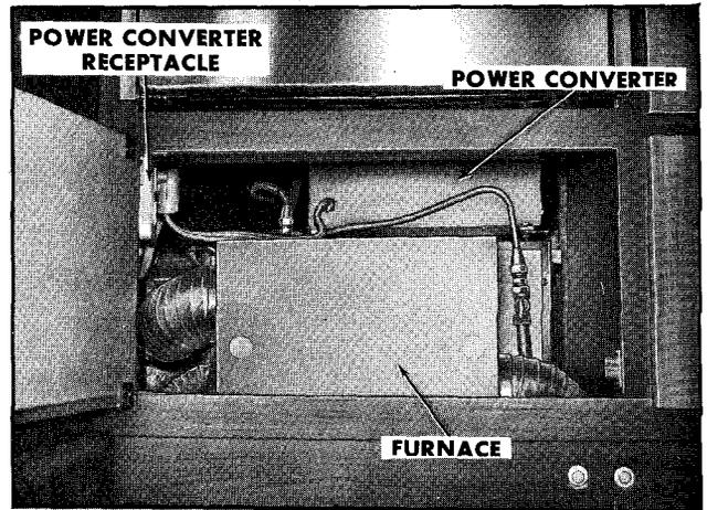
Figure 3—Converter Location (Model ZEO6582)
