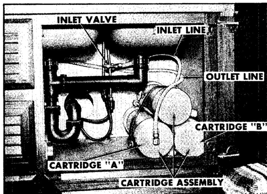
Figure 2—Water Treatment Unit Cartridge Location
